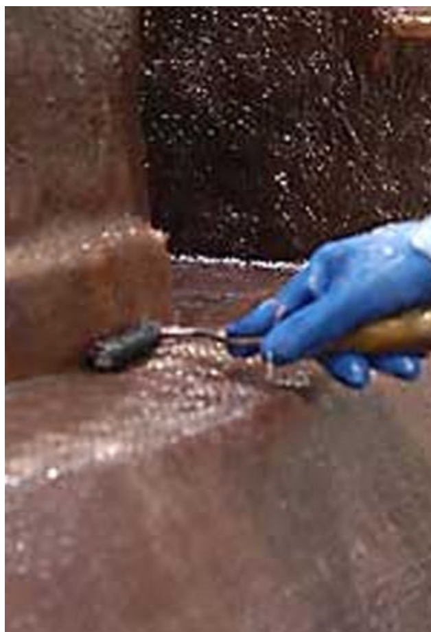
Hand lamination ensures the strongest hull and best ratio of resin to fiberglass.
